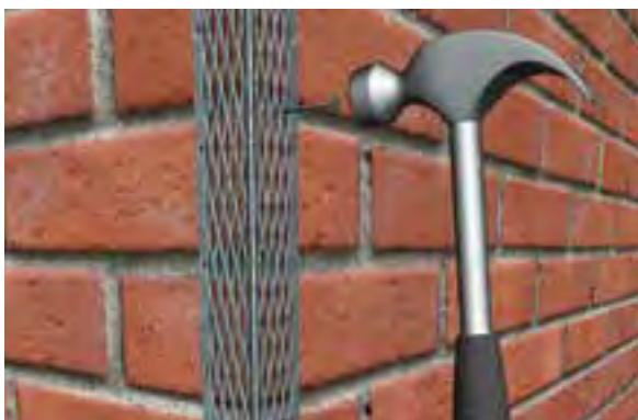
■ NAILING INTO THE MORTAR ON MASONRY WALLS
