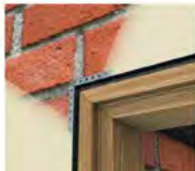
■ DOOR JAMB WITH SHADOW EFFECT USING R50
