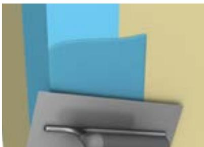
Apply second coat to a width of approximately 120mm. Allow to dry, then remove any excess and lightly sand if necessary.
