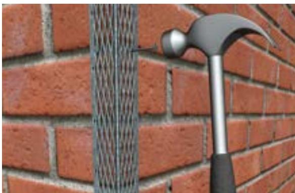
■ NAILING INTO THE MORTAR ON MASONRY WALLS
