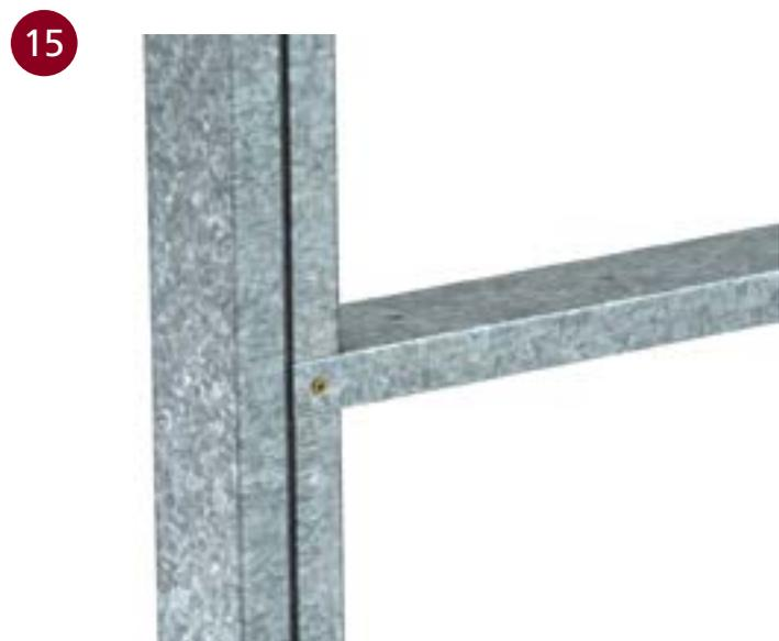
■ NOGGING TRACK FIXING DETAIL AT MAXIJAMB
