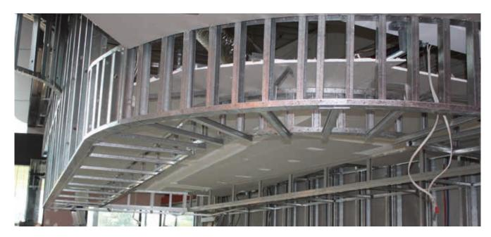
The construction of box type bulkheads to conceal services can be designed into a wall or ceiling, and are sometimes found necessary on site because:
